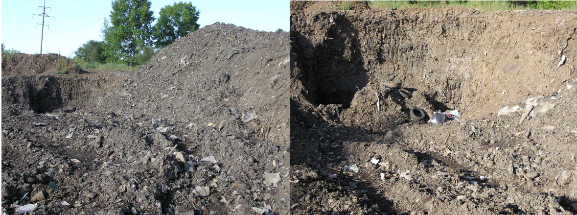
Figure 5, 6. Margin of landfill disturbed by scrap diggers.
